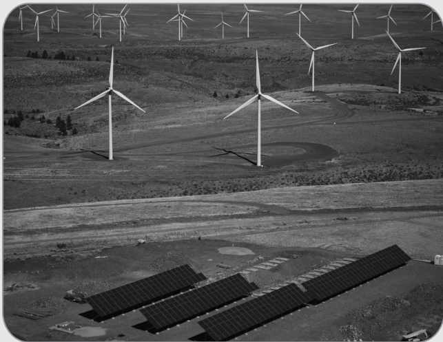
A solar-power generating plant operates alongside the 127 turbines at PSE's Wild Horse Wind and Solar Facility in Kittitas County.
