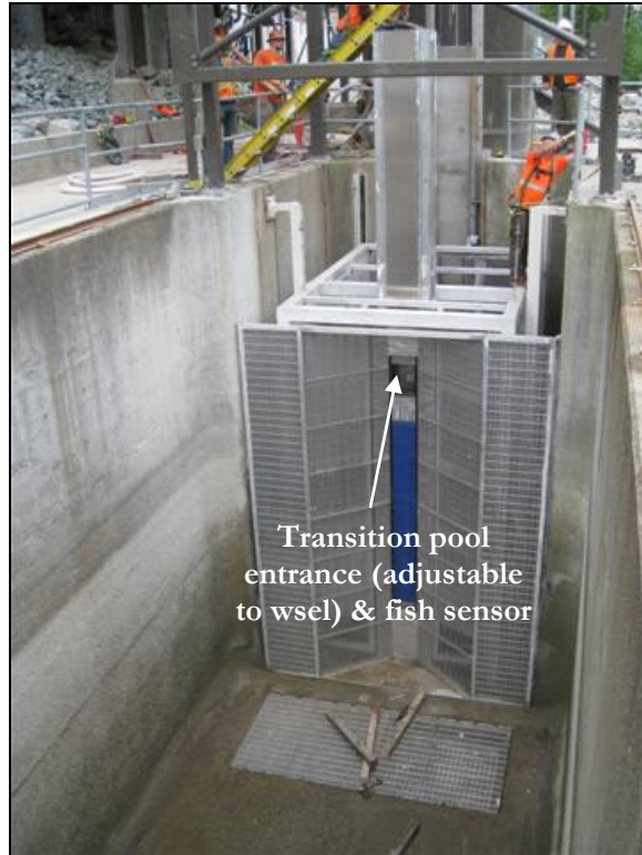
Figure 10. Transition pool entrance and fish sensor.
