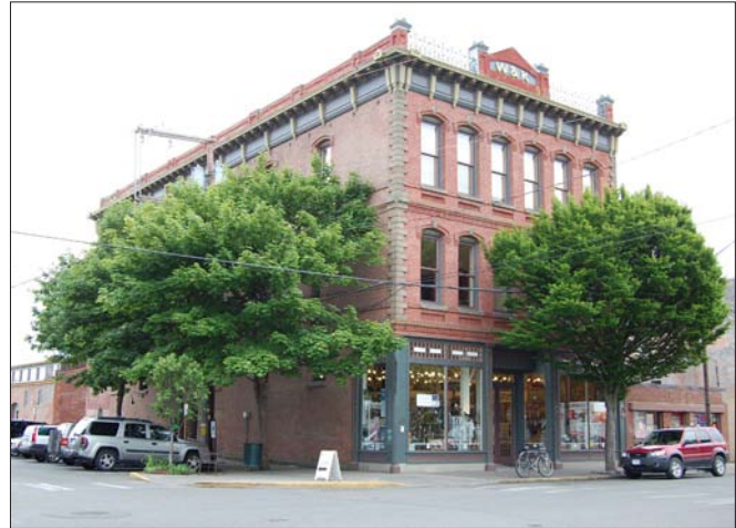
Waterman & Katz Building in Port Townsend
