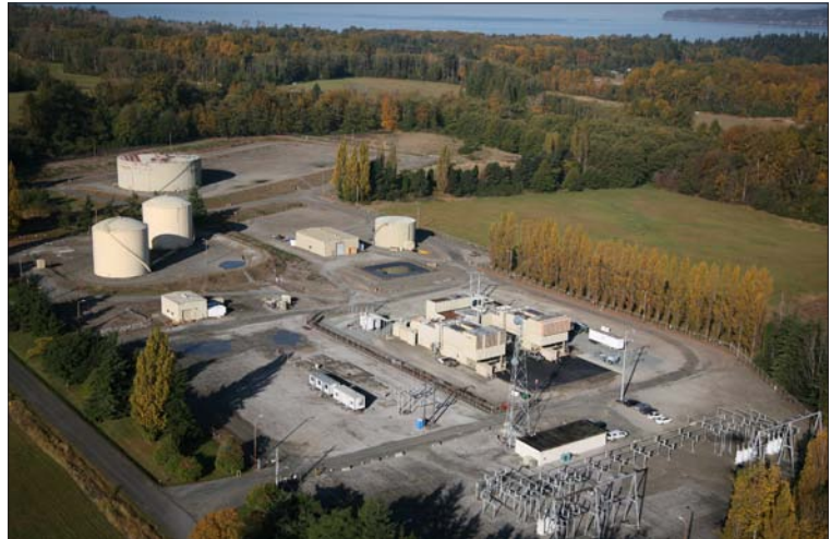
Whitehorn Generating Station
