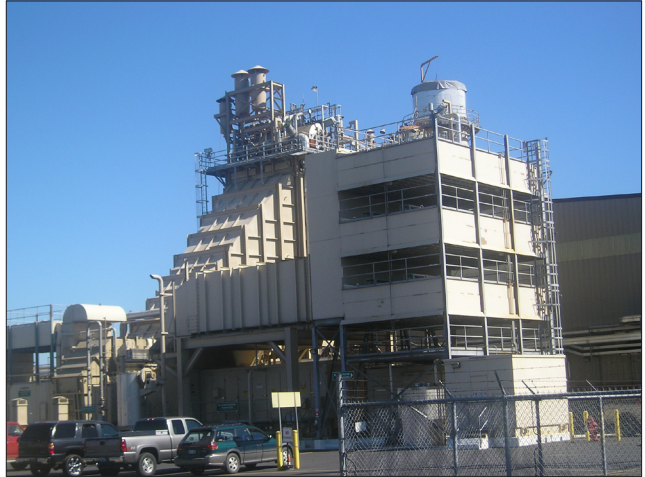
Sumas Generating Station
