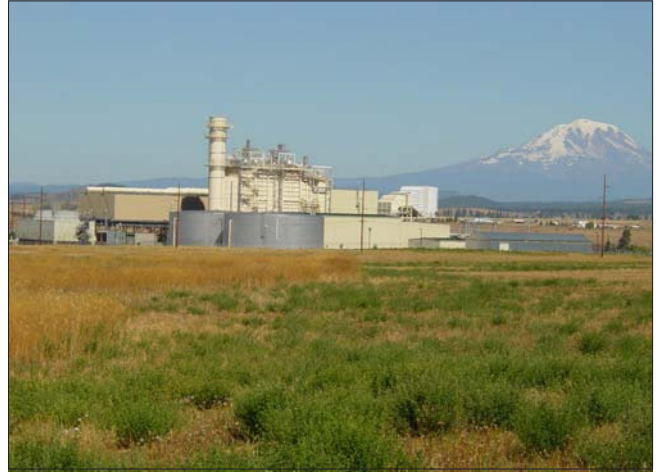
Goldendale Generating Station
