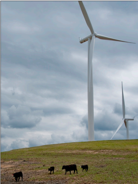
Wind power and agriculture go well together. More than 99 percent of the land at PSE's Lower Snake River Wind Facility remains available for farming and livestock grazing.
