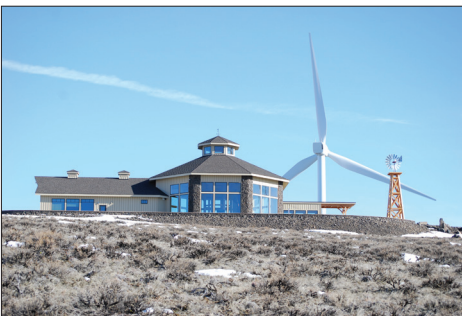
The Renewable Energy Center allows visitors to explore the latest technologies in wind and solar power, and learn about the Kittitas Valley.
