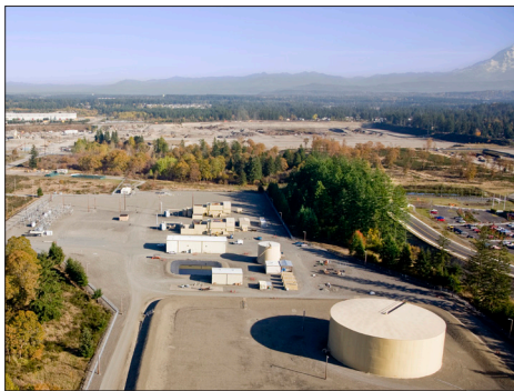
Frederickson Generating Station
