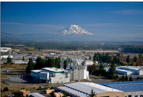
Frederickson 1 Generating Station
