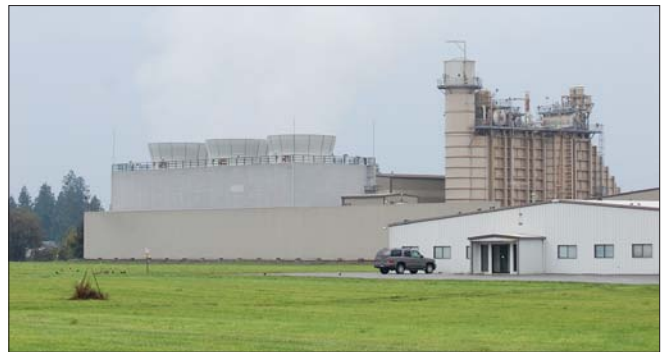
Sumas Generating Station
