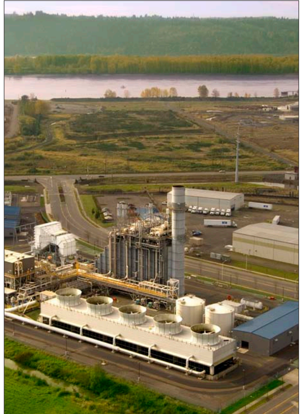
Mint Farm Generating Station
