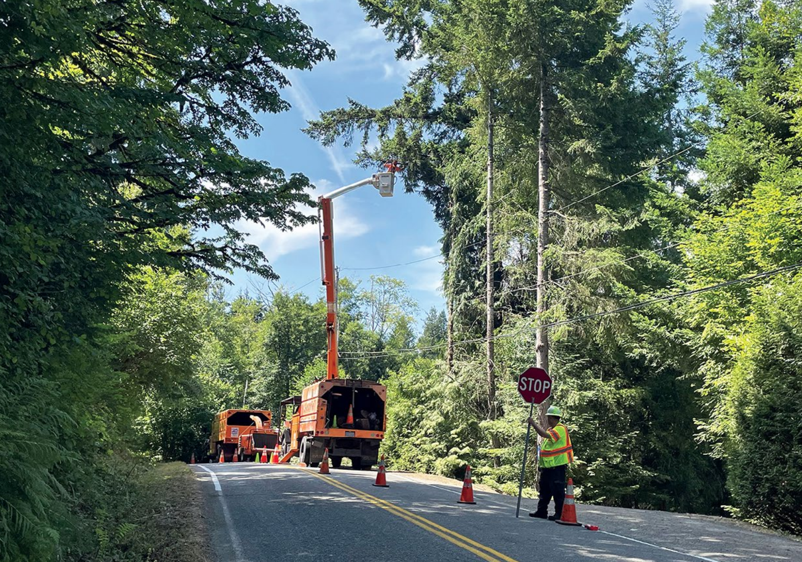
Crews trim back vegetation near power lines on Bainbridge Island
