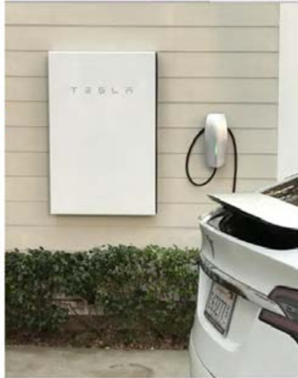
7 kW/14 kWh residential customer-sited lithium-ion battery.
