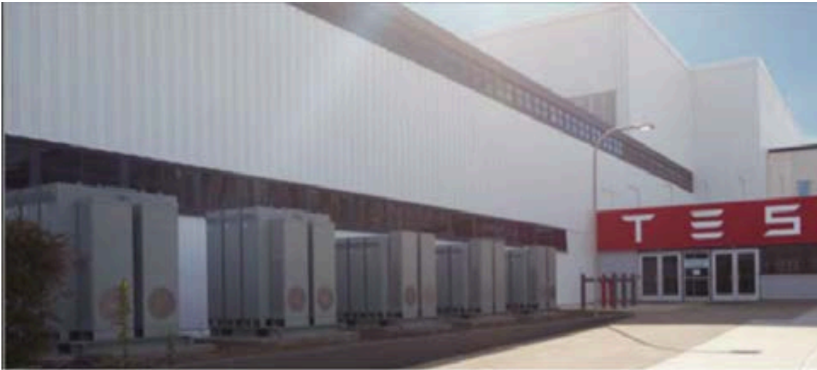
1 MW/2 MWh customer-sited lithium-ion battery.
