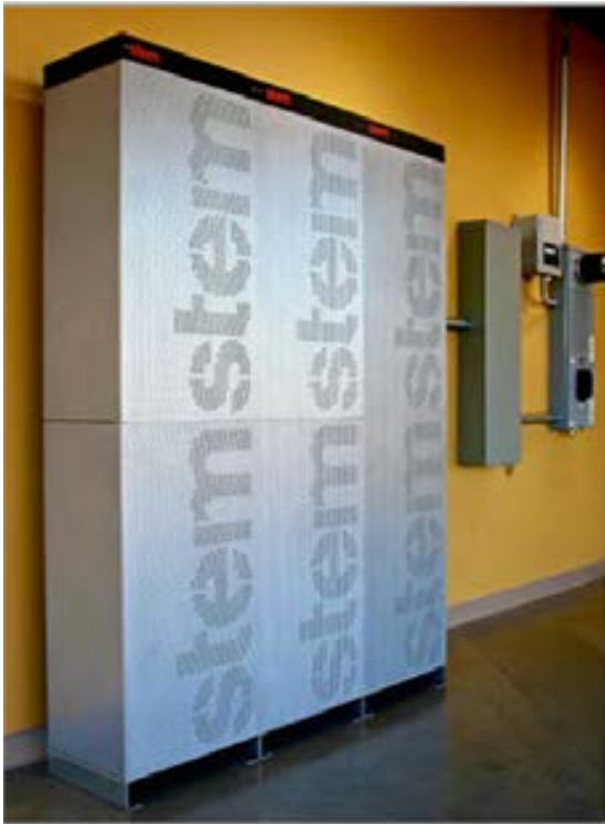
54 kW/54 kWh commercial customer-sited lithium-ion battery.
