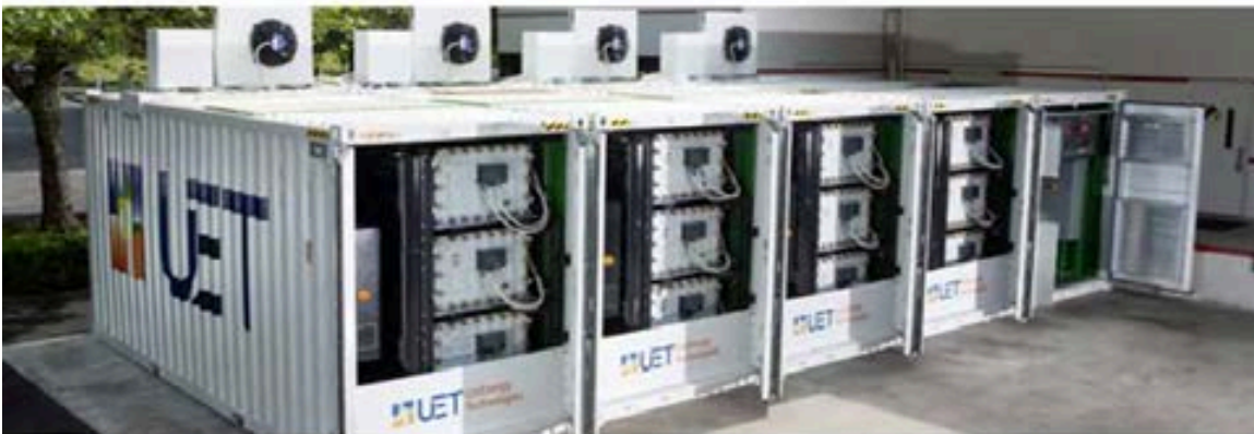
1 MW/3.2 MWh distribution-connected vanadium redox flow battery.
