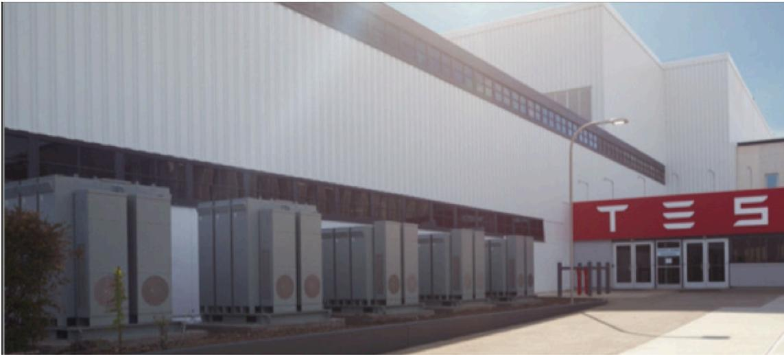
1 MW/2 MWh customer-sited lithium-ion battery.
