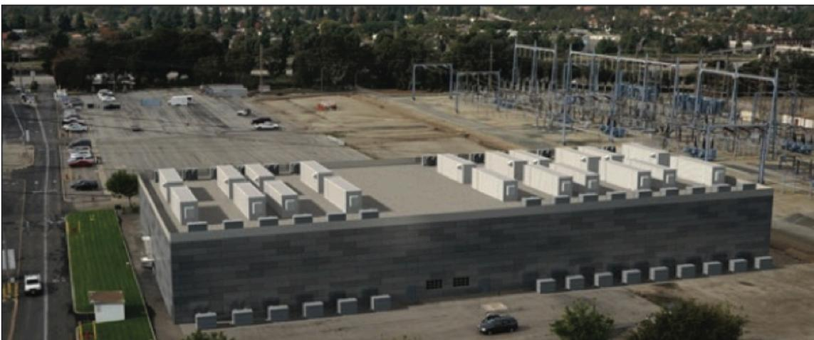
Proposed 100 MW/400 MWh transmission-connected battery.
