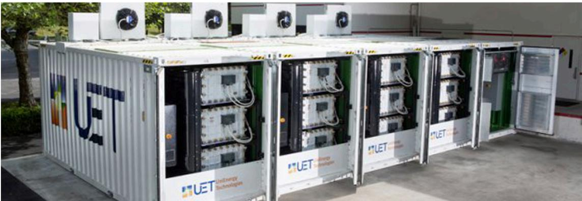
1 MW/3.2 MWh distribution-connected vanadium redox flow battery.
