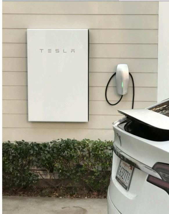
7 kW/14 kWh residential customer-sited lithium-ion battery.
