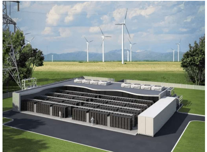
Battery Energy Storage System (aka BESS)
