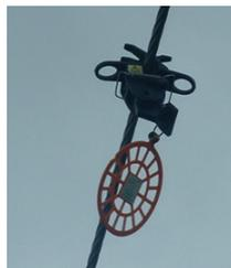
Line markers increase visibility of power lines to reduce the potential for collisions.
