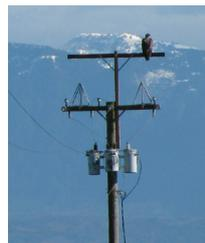
Equipment covers include bushing covers, cut out covers, and covered jumpers, which reduces the risk of bird electrocution on equipment poles.
