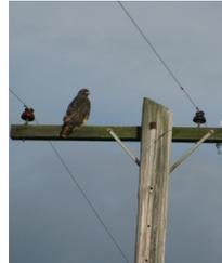
Perch deterrents help move birds from unsafe parts of the crossarm to a safer perch with wider spacing between conductors.
