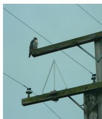
Perches provide a safe place for birds to perch on preferred poles away from electrical equipment.
