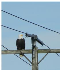
Bird guards allow birds to perch safely on utility poles by covering energized conductors and providing sufficient spacing between conductors.
