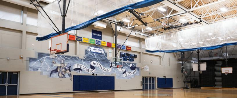
Sensors in the gym at Squalicum High School automatically turn off lights when the space isn't in use. Additionally, lighting controls are programmed in three distinct sections of the gym so that one, two or all three sections can be lit as use of the space demands.
