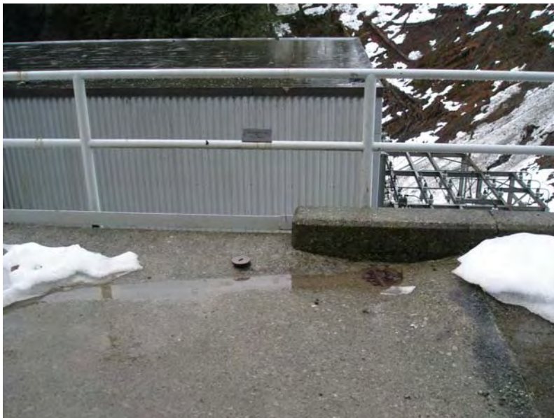
Photo 2. The drain at the Upper Baker Powerhouse. The drain collects runoff from a small concrete pad at the entrance to the Powerhouse and discharges to the Upper Baker Tailrace (Baker River). A permanently capped, unused fill port is located to the left of the drain.
