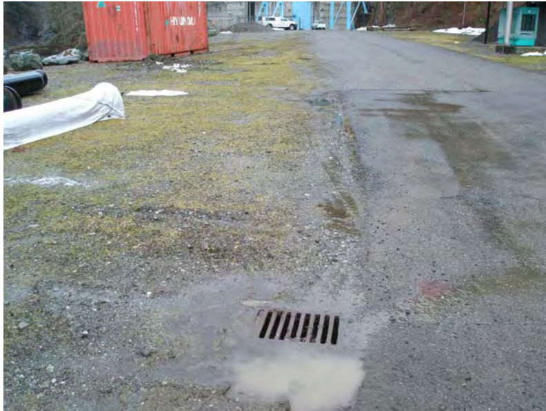
Photo 3. View looking northeast at Catch Basin "B". Catch Basin B collects surface runoff from a portion of the roadway and adjacent gravel area northeast of the catch basin (see Figure 6). The outfall for Catch Basin B drains to the Lower Baker Tailrace (Baker River).
