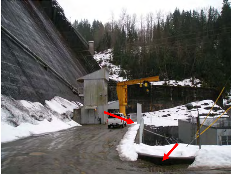
Photo 1. View looking southwest at Catch Basin “A” (right arrow). A small drain is located in the background (left arrow, see photo 2). The drain discharges to the Upper Baker Tailrace (Baker River).
