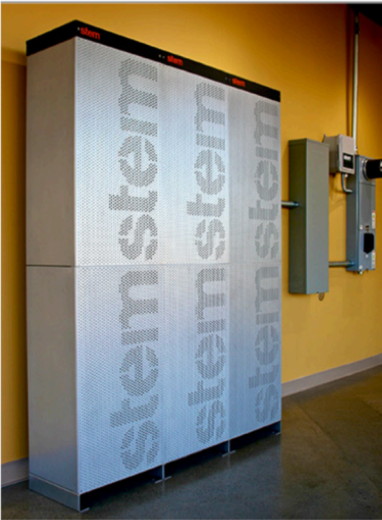
54 kW/54 kWh commercial customer-sited lithium-ion battery.
