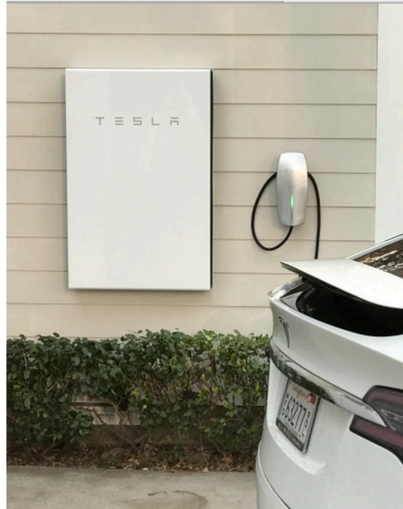
7 kW/14 kWh residential customer-sited lithium-ion battery.
