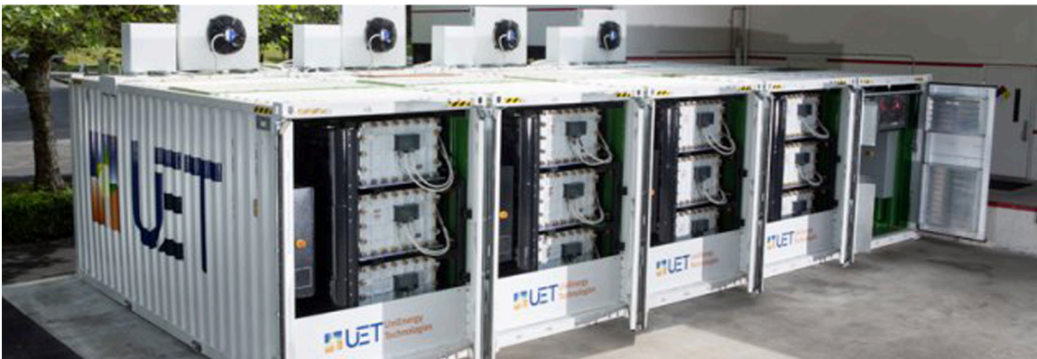
1 MW/3.2 MWh distribution-connected vanadium redox flow battery.
