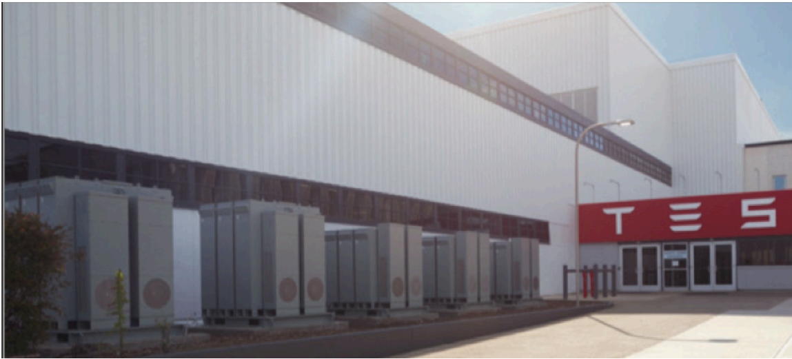
1 MW/2 MWh customer-sited lithium-ion battery.
