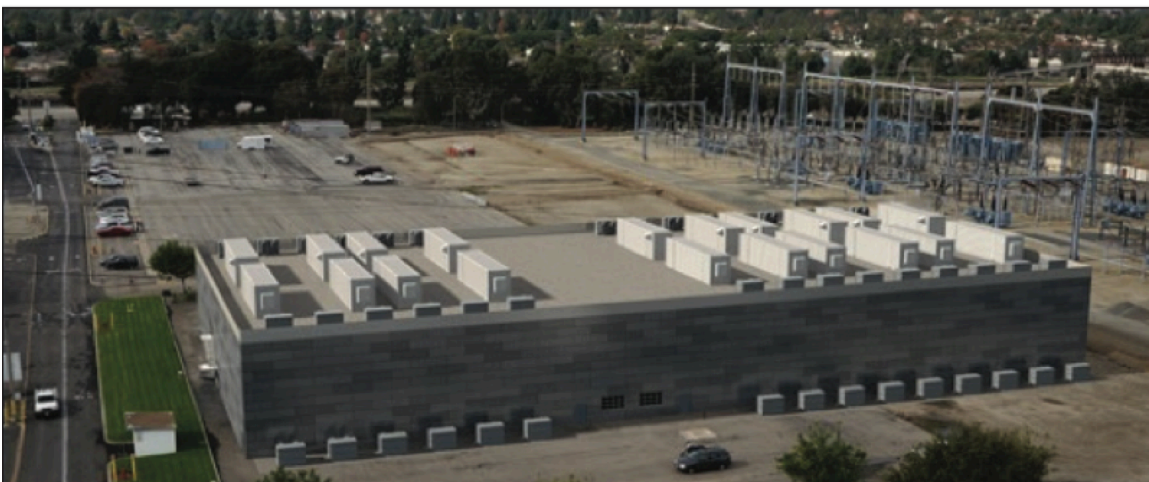
Proposed 100 MW/400 MWh transmission-connected battery.
