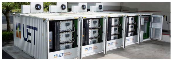
1 MW/3.2 MWh distribution-connected vanadium redox flow battery.
