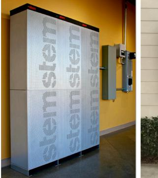
54 kW/54 kWh commercial customer-sited lithium-ion battery.
