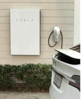
7 kW/14 kWh residential customer-sited lithium-ion battery.
