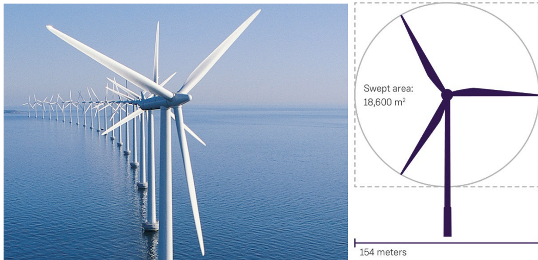
Figure 2-1. Offshore 6 MW Wind Turbines and Diagram
