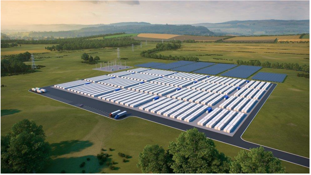
An artist rendering of a 56 megawatt energy storage system, with iron-air battery enclosures arranged next to a solar farm. Image courtesy of Form Energy.
