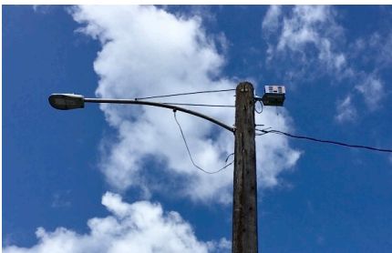
Device attached to light pole
