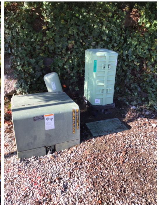
Pedestal device (right) next to a pad-mounted transformer
