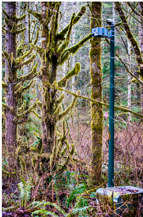
Pole device in area with underground electric service
