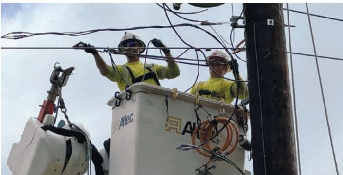
Upgrading the Poulsbo grid
