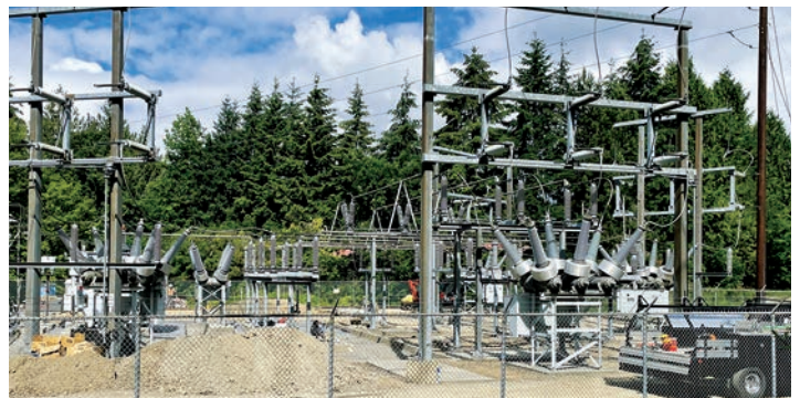
Port Madison substation construction on Bainbridge Island
