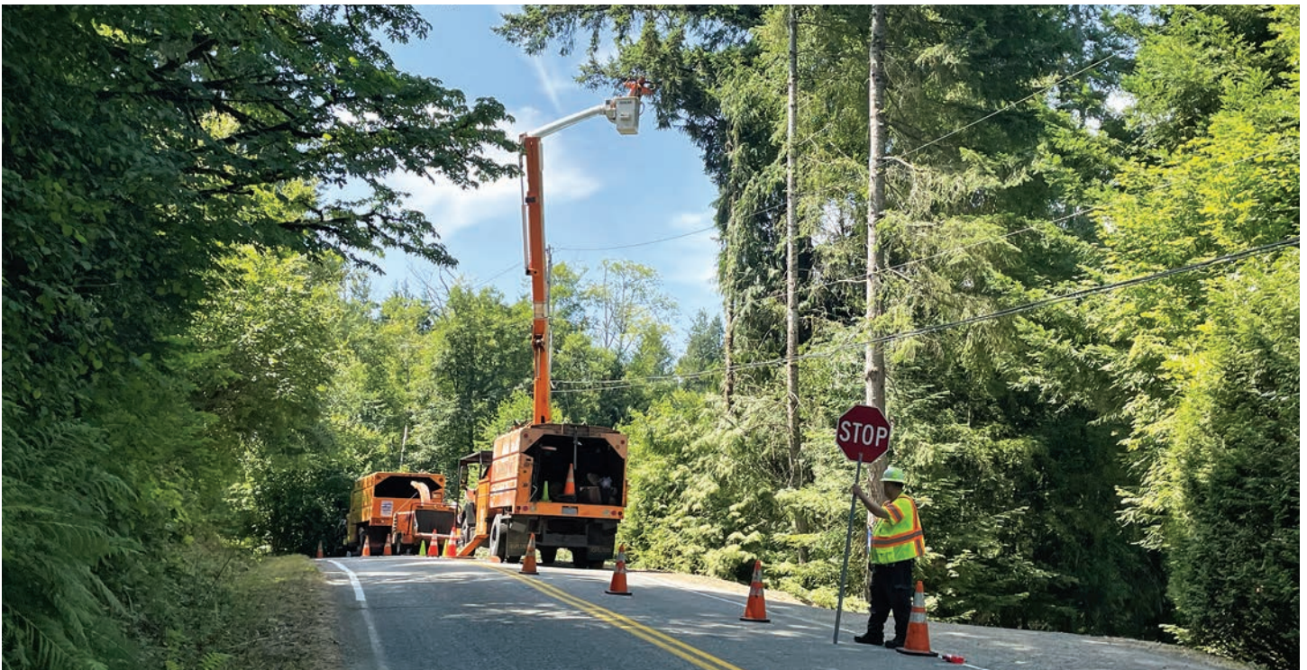
Tree trimming on Hidden Cove Road
