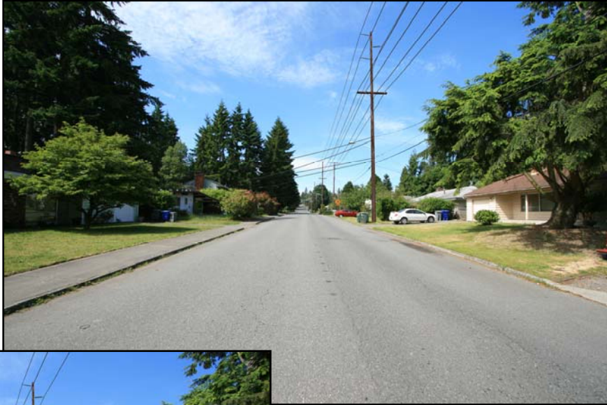
Distribution with transmission overbuild
