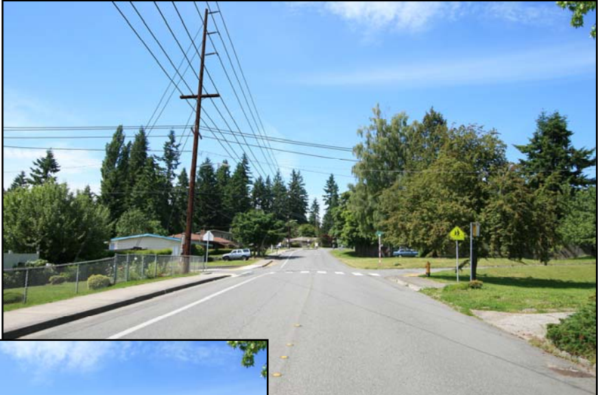
Distribution with transmission overbuild
