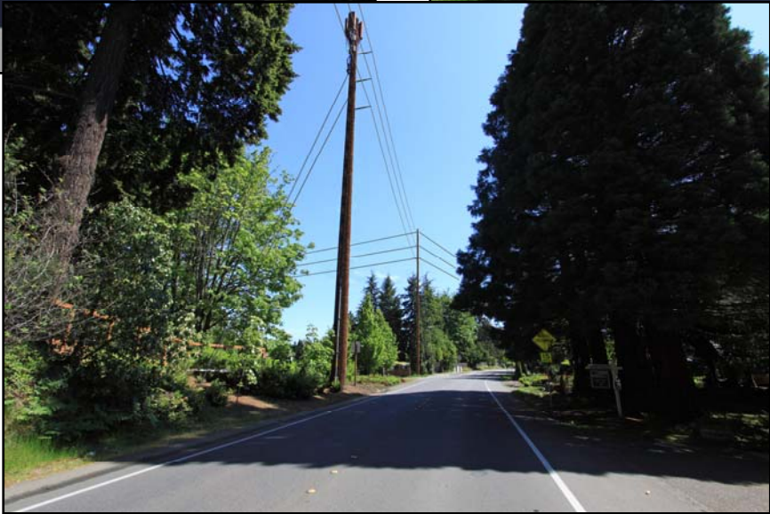
Transmission with underground distribution
