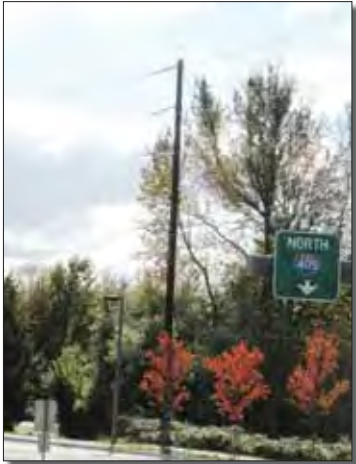
Single-circuit 115 kV wood pole without distribution underbuild
