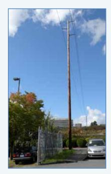
Example pole with average heights ranging from 65 feet to 75 feet depending on topography and span length.
