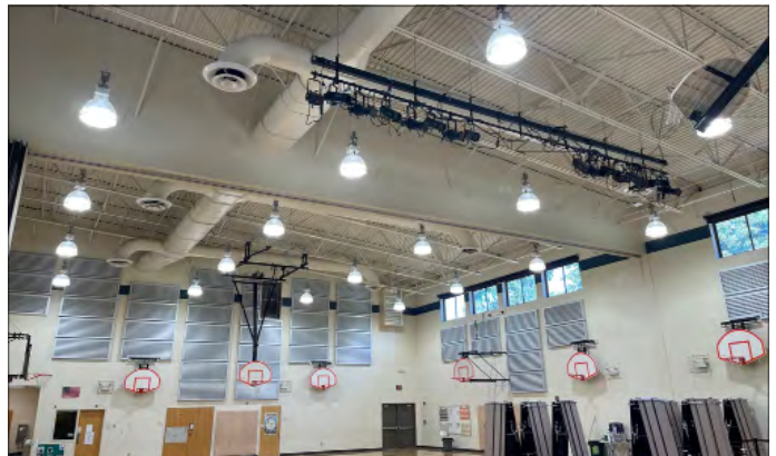
An LED lighting retrofit project in the gym at Lake Hills Elementary.
