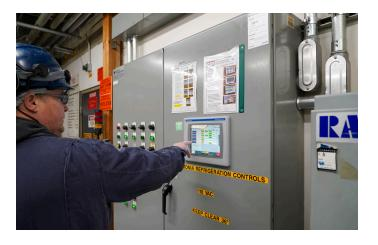
Installing variable-frequency drives on condenser cooling fans helped stabilize energy usage for refrigeration, resulting in large energy savings.
