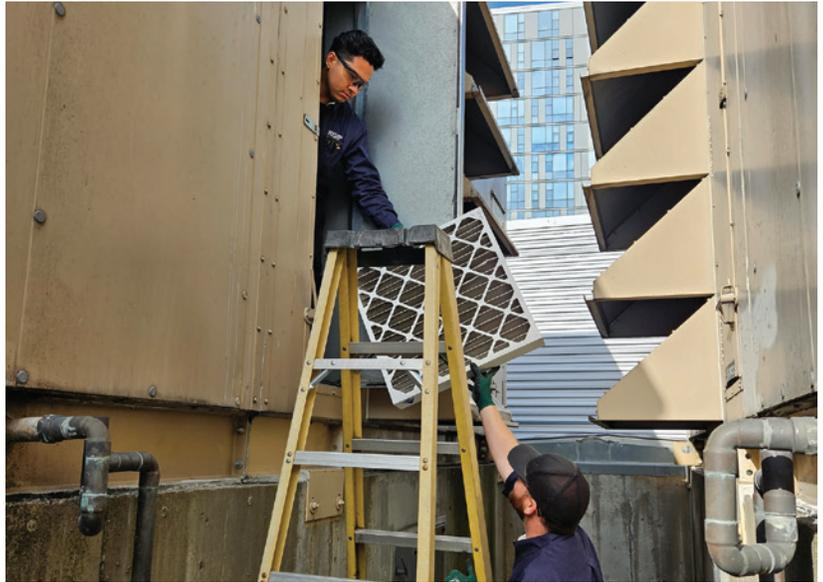
Simple practices like regularly changing air filters have a huge impact on overall HVAC efficiency — or inefficiency if they’re not done. This critical link is a focus of the Accelerator, and KGIP makes it a high priority.
