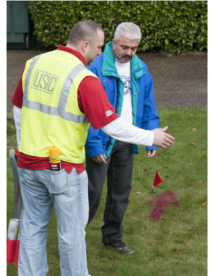
A representative from PSE's locate service shows a customer where underground utilities are located on his property.
